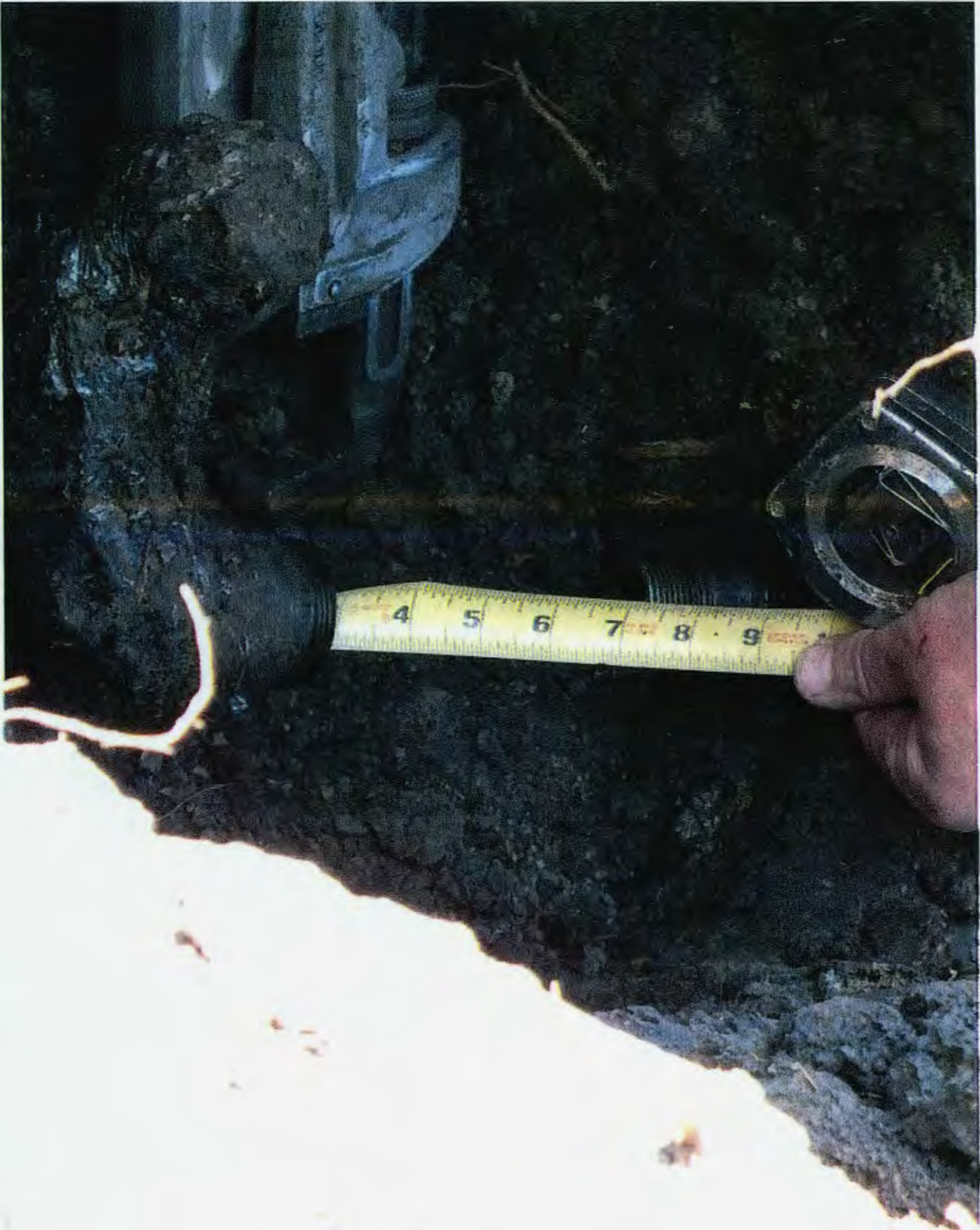
EXHIBIT 9 Service Line Pulled from Compression Fitting
