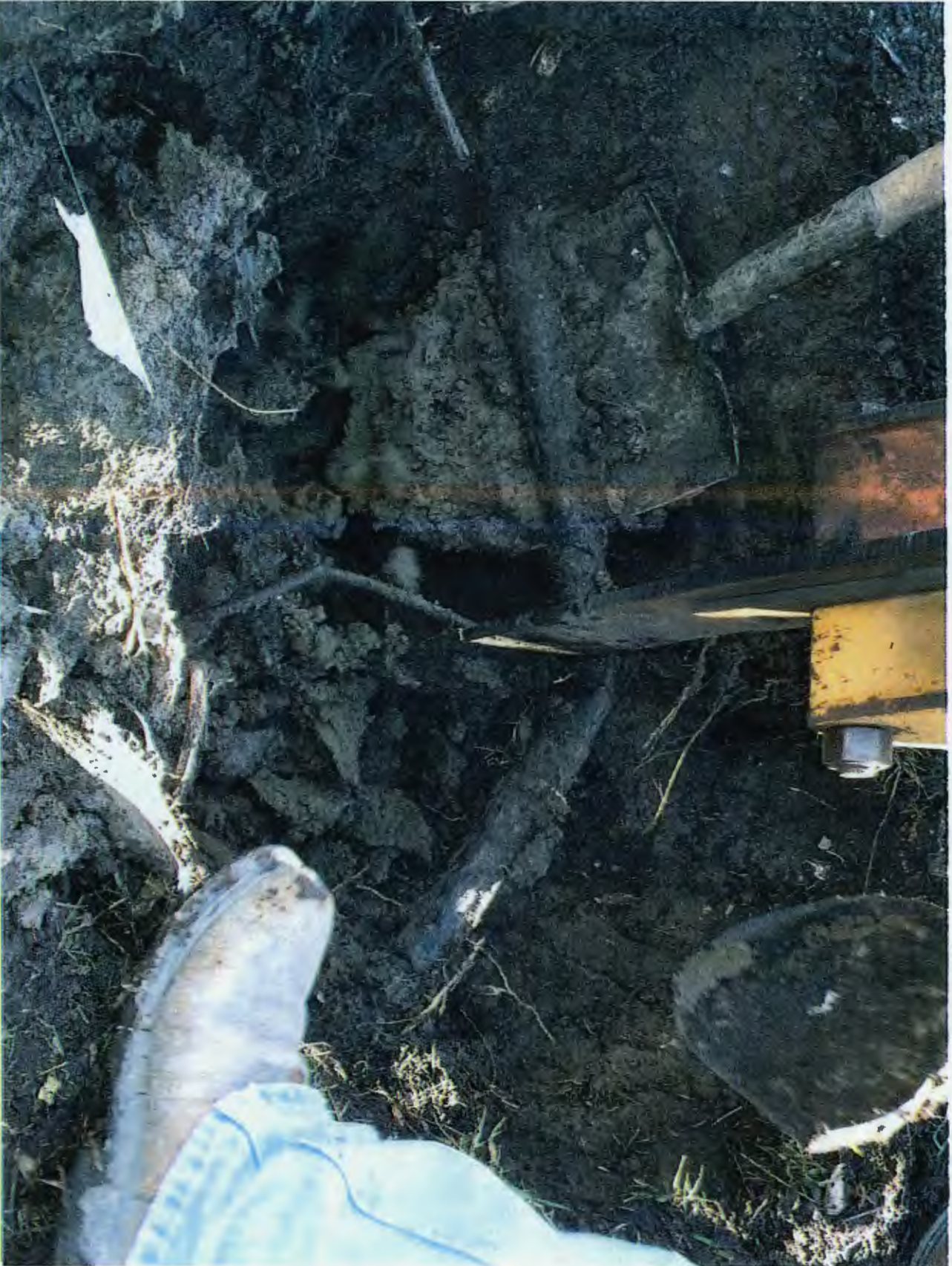
EXHIBIT 5 Service Line Damage Caused by Vibratory Plow
