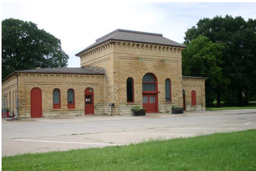
Park House in Wellington was used as a community center and now houses the Panhandle Railroad Museum.
