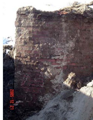
The outside wall of the coal tar well. This kind of brick construction was typical of underground structures at a manufactured gas plant.
