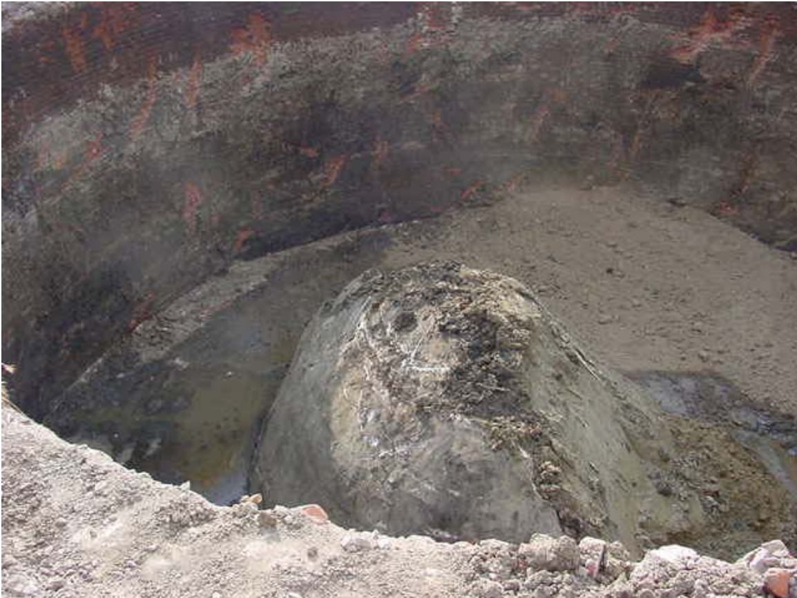
An excavated gas holder tank in Kansas City. In this picture is the “dumpling,” made of bedrock or concrete, usually left in the holder tank in order to support the gas holder framework and piping.
