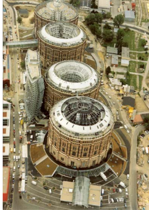
These gasometers in Vienna were used until 1984, and have since been converted to retail, office, and living space.
