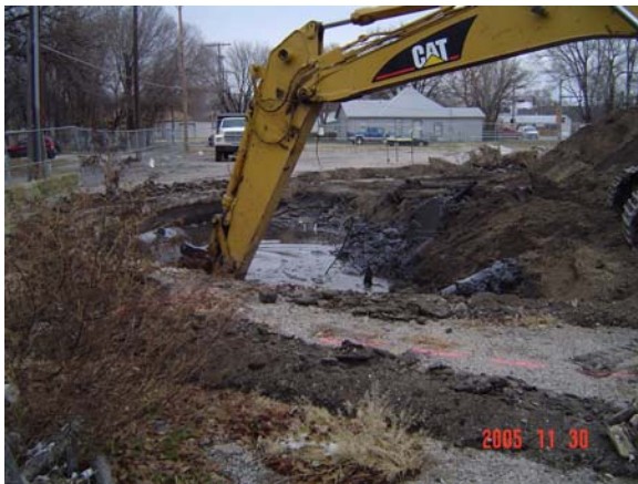
Removing the contents of the gas holder tank at the former manufactured gas plant in Manhattan. The contents are primarily water, woody debris, soil, and hard-parts refuse.
