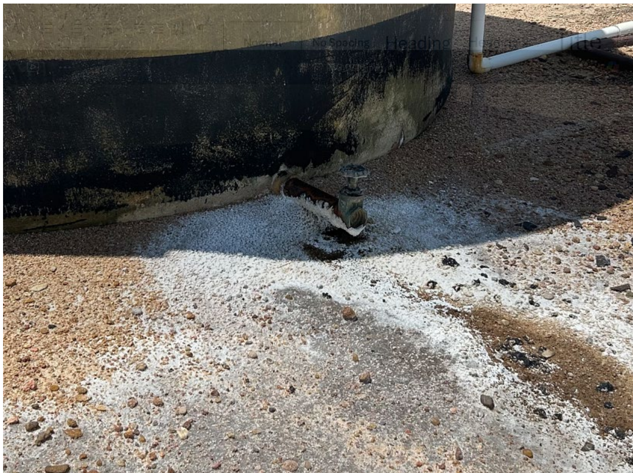
Clinton Production, Inc. #5585 D J Moore Tank Battery Sec. 36-24-9W, Reno Co. Photo showing leak from saltwater tank. Date: 6-25-2025
