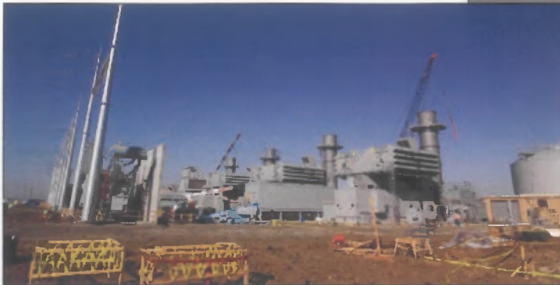
Overview of Emporia Energy Center construction.
