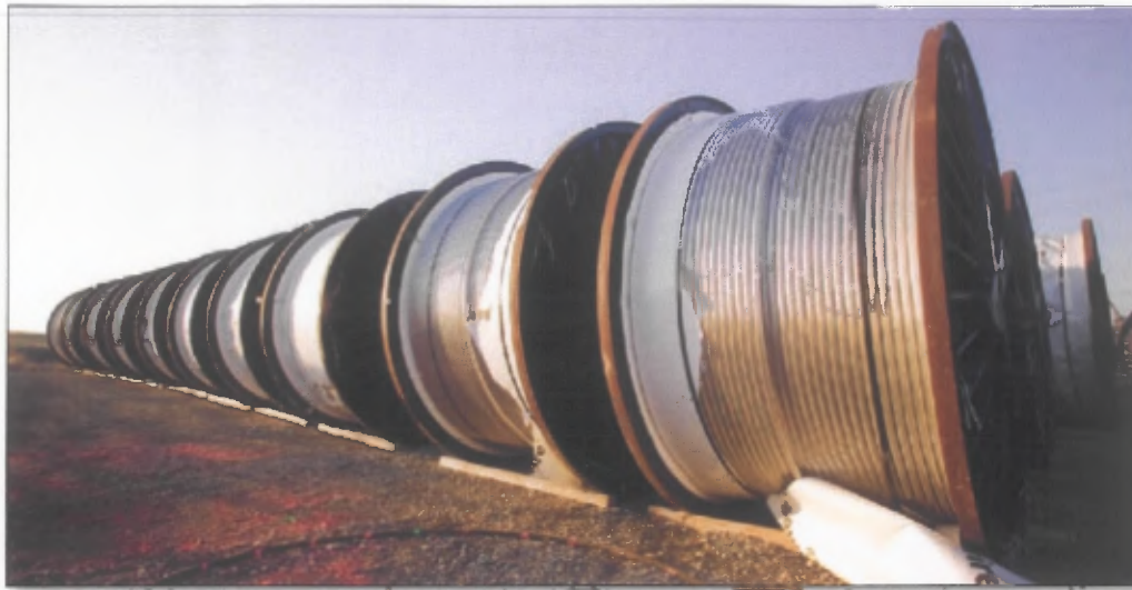
Reels of wire at Gordon Evans Energy Center that will be used for the new 345 kV line from Wichita to Hutchinson, and then to Salina. Construction is expected to be complete by late 2009.
