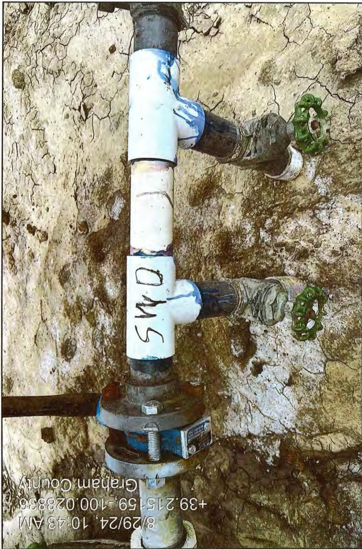
Above: The opposite side of the manifold shows that one line is labeled "SMD", while the other is unlabeled.
