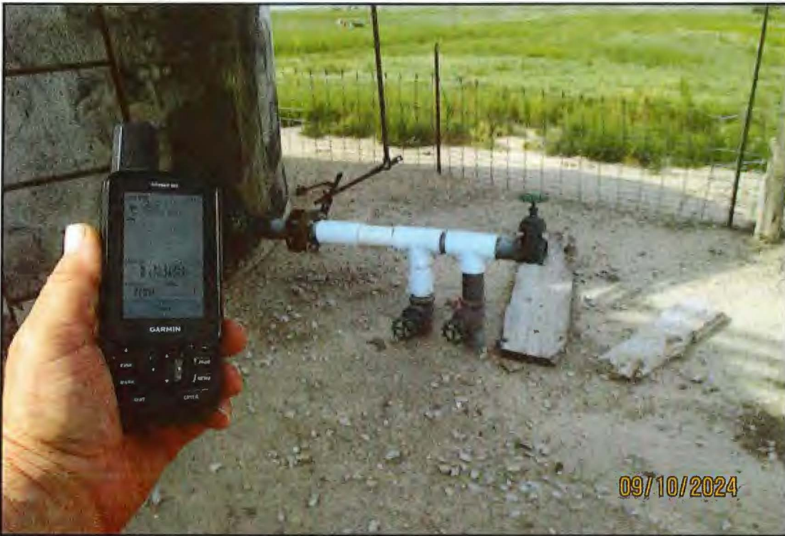
Above: View of the brine tank located at the tank battery. The brine tank is located @ 39.27303N & -100.28703W. Leo: NE-NW-SE-NW/4 of section 13-9-27W. 3782' FSL & 3411' FEL. At the time of inspection the outside (vertical) 3" valve was in the closed position. The inside (vertical) valve was in the open position. The brine tank fluid level was slightly above the halo valve exit line. The tank float was approximately 5' above the fluid level.
