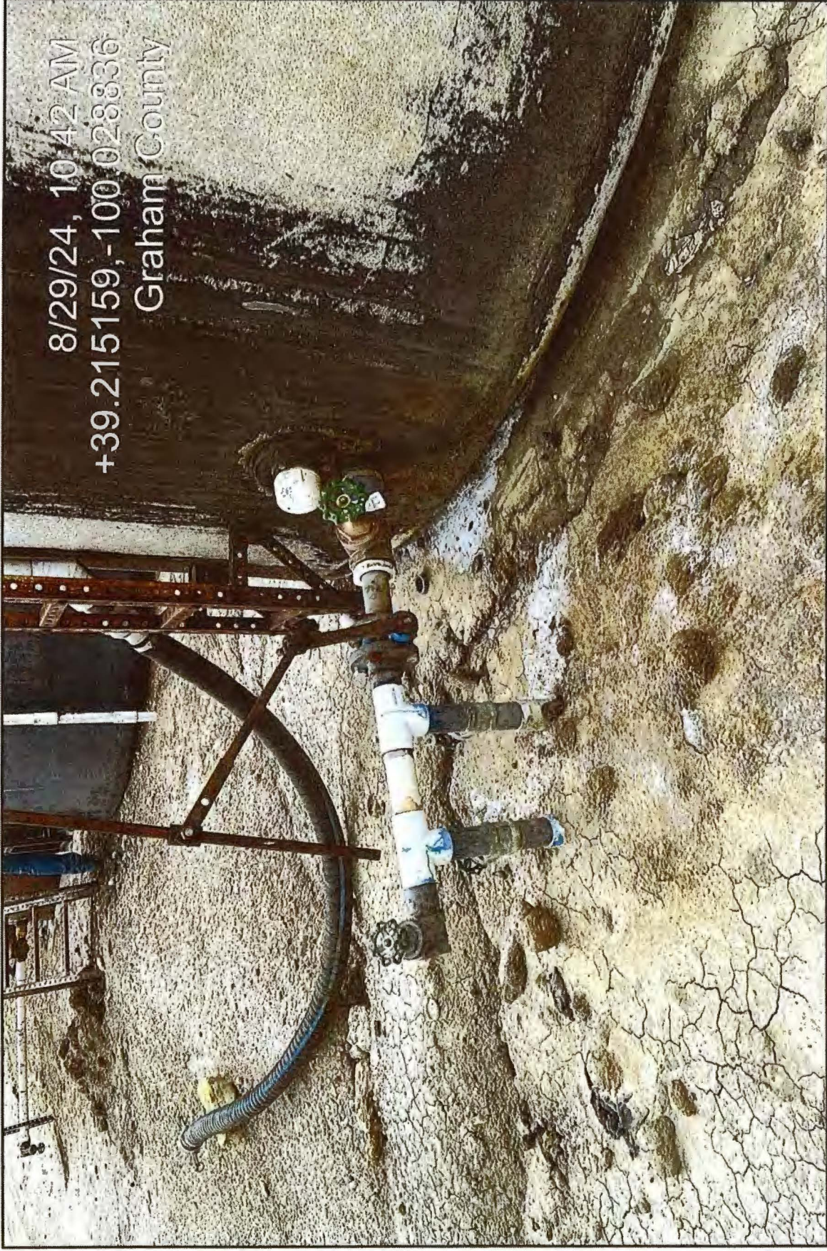
Above: The brine tank is equipped with a manifold system after the main gate valve and halo valve. The lease has a single permitted disposal well, while there are two brine line outlets at the tank.
