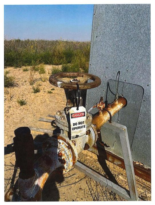
Date: 10/8/2024 Operator: C & R Petroleum Co. Well Name: Sandifer 1 Legals: SE-NW-NW-SW section 30-34s-34w Seward County Description: Meter run showing closed and tagged downstream valve.
