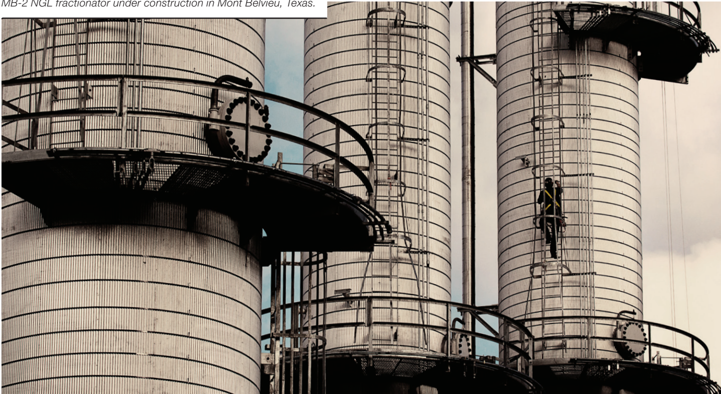
MB-2 NGL fractionator under construction in Mont Belvieu, Texas.
