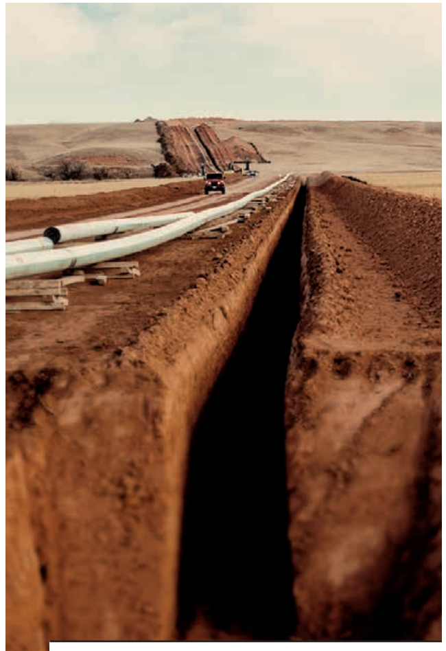
Bakken NGL Pipeline construction in northeast Wyoming.
