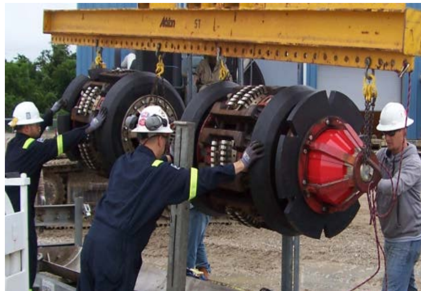
36-inch Magnetic Flux Axial Flaw Detection In-Line Inspection tool being loaded into Line X
