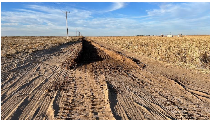
Photo #15 Looking north at the northern portion of the excavated North-South access road. Excavation was to 2 feet.
