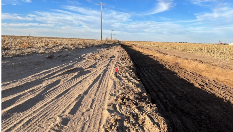
Photo #16 Looking north at the west side of the northern portion of the excavated North-South access road. Excavation was to 2 feet. An underground electric line is marked by the red flags.
