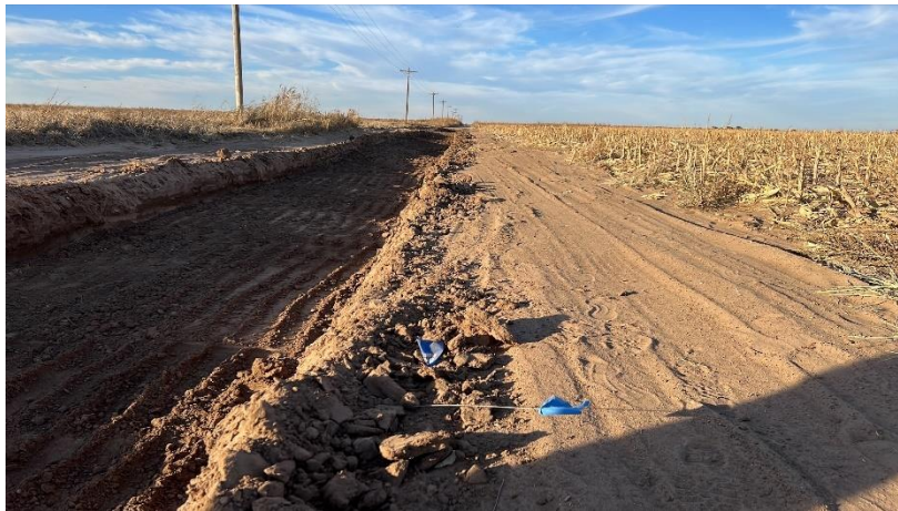
Photo #17 Looking north at the east side of the northern portion of the excavated North-South access road. Excavation was to 2 feet. An underground water line is marked by the blue flags.
