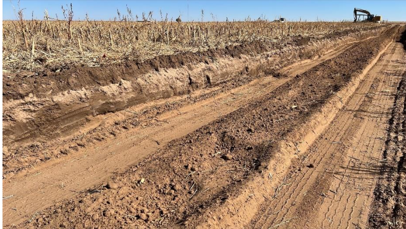
Photo #13 Looking northeast eastern portion of the East-West access road to A3 excavated to 4 feet.
