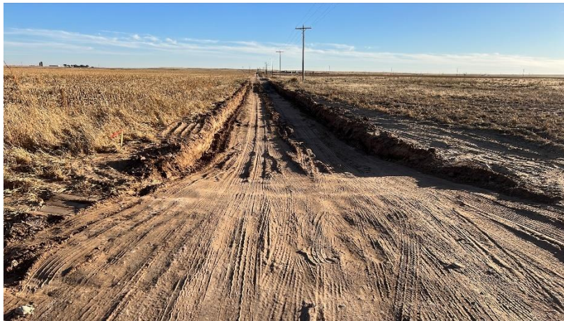
Photo #14 Looking south at the southern portion of the excavated North-South access road. Excavation was to 2 feet.
