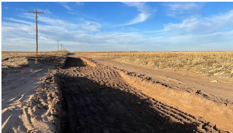
Photo #18 Looking north at the northern portion of the excavated North-South access road. An underground electric line and petroleum line cross the road in the unexcavated area at the left-center of the photo.
