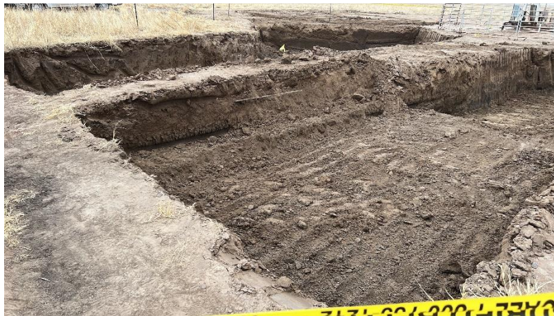
Photo #8 Looking southeast at the two portions of Excavation Area E (Webb A3). A buried electrical line is located within the un-excavated area. Excavations are four feet deep. The northern portion of Excavation Area D and located to the top right (south) of the photo.
