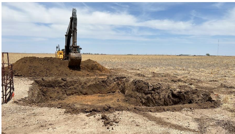
Photo #3 Looking north at Excavation Area B (Webb A1). Excavation will be six feet deep and will be over-excavated to 10 feet.
