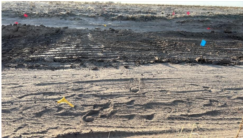
Photo #20 Looking west at the northern portion of the excavated North-South access road. An underground petroleum line crosses the road in the unexcavated area marked by the yellow flags.
