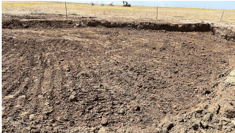
Photo #5 Looking northwest at Excavation Area C (Webb A3). Excavation is two feet deep.
