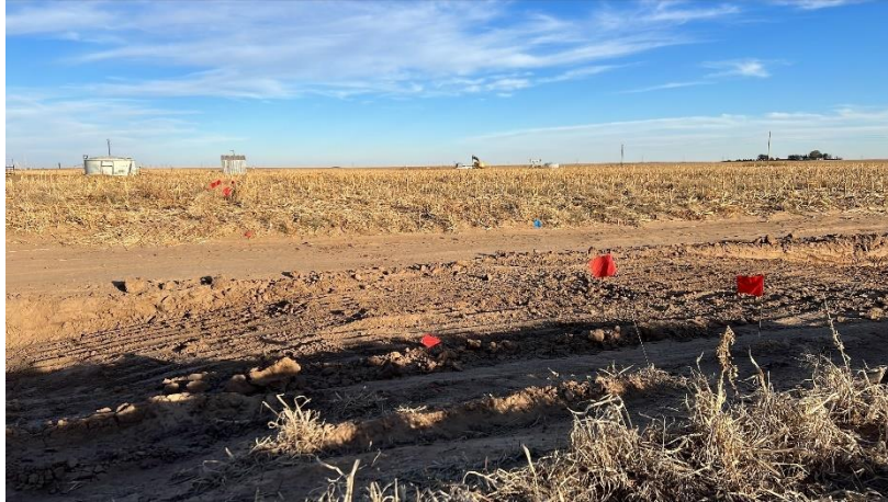
Photo #19 Looking northwest at the northern portion of the excavated North-South access road. An underground electric line crosses the road in the unexcavated area marked by the red flags.
