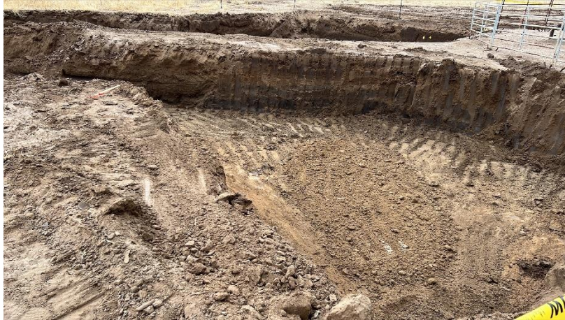
Photo #7 Looking east at the two northern portions of Excavation Area D (Webb A3). A buried electrical line is located within the un-excavated area. Excavations are six feet deep.
