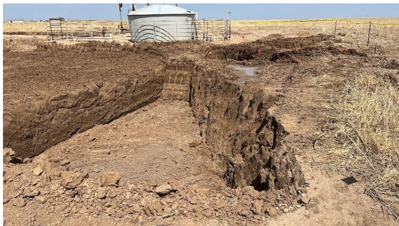
Photo #6 Looking east-northeast at the three southern portions of Excavation Area D (Webb A3). Buried electrical lines are located within the un-excavated flagged areas. Excavations are six feet deep and will be over-excavated to 10 feet. Excavation Area C is located to the left (north) of the photo.
