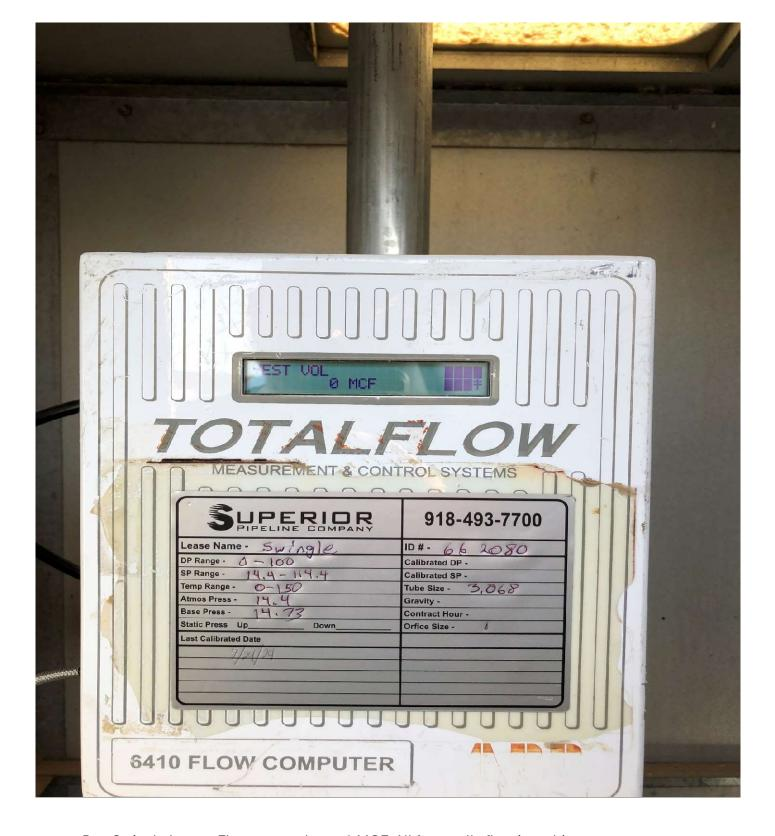
Ben Swingle Lease, Flow meter shows 0 MCF. All four wells flow into this one meter.
