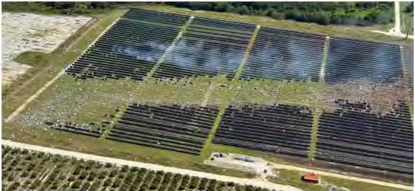
Tornado damage to solar plant in Florida
