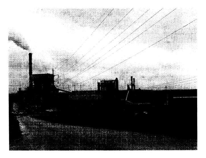
Lawrence Energy Center presently has three units that are reliable base-load units. Unit 5 is to the far left, with smoke coming out the stack. Unit 4 is to the far right of the photo. Housed in the building in the middle are units 1, 2 and 3, with 3 being the only one running. Units 1 and 2 have been retired in place.
