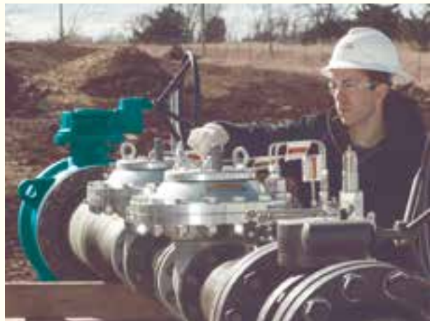
Oklahoma Natural Gas completed a pipeline project to supply the Stillwater Energy Center with efficient natural gas.
