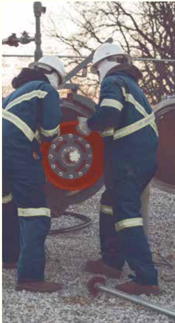
Employees near Sapulpa, Okla. insert a “pig” as part of procedures to inspect a pipeline. Pigs are used to perform various maintenance tasks and inspections on certain pipelines.
