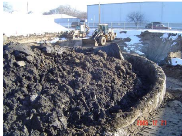
Excavated material from the site placed in the gas holder tank to soak up water contaminated with coal tar. The contaminated material was removed and properly disposed of at a hazardous waste disposal facility.
