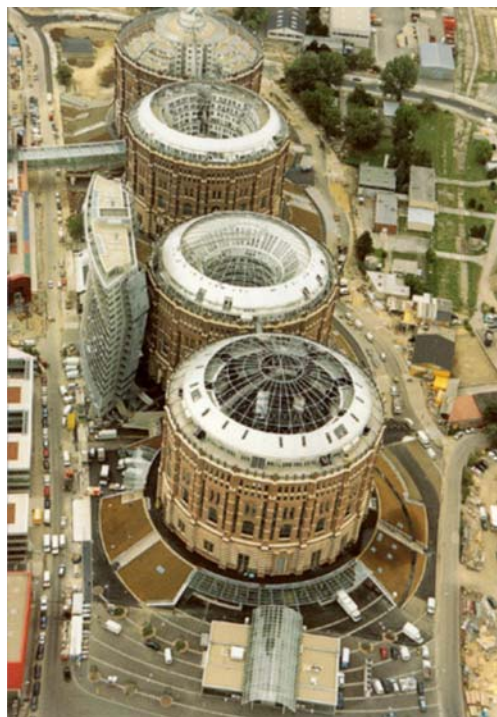
These gasometers in Vienna were used until 1984, and have since been converted to retail, office, and living space.
