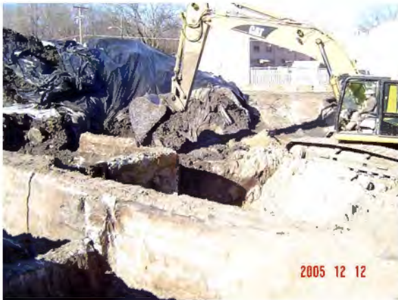
Excavation revealed underground foundations and structures. These were left in place when clean fill was installed.
