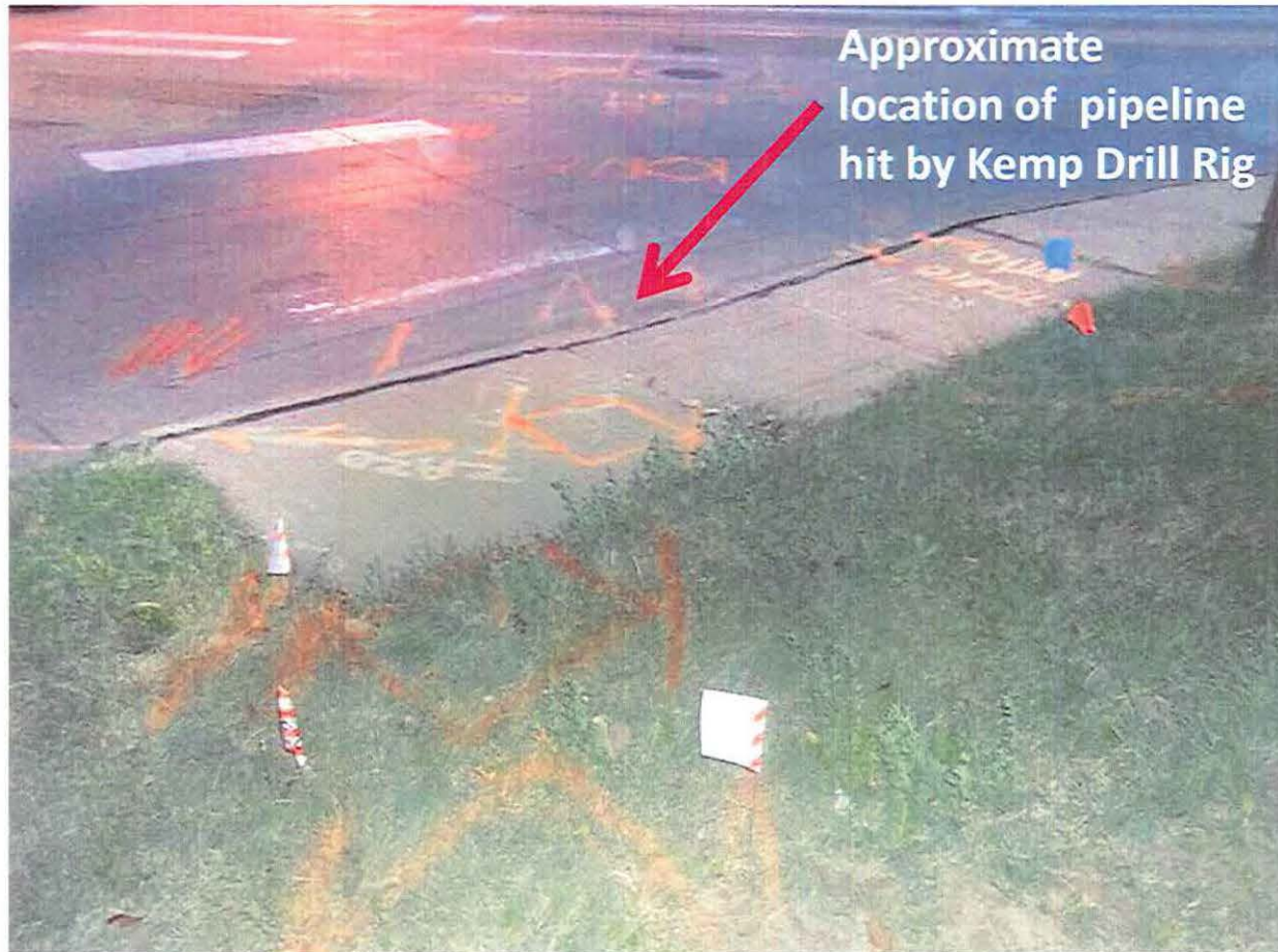
Property of United States Infrastructure Corporation Photo taken on 10/12/2016 7:27:12 AM
