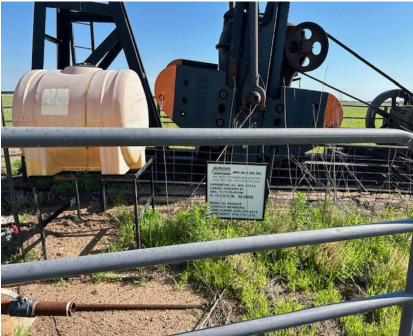
Well is fully equipped but has failed to operate.
