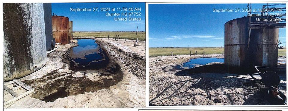
Horchem A Tank Battery GPS: 38.72105, -100.20858 3166' NSL & 5169' WEL NW SW SW NW 27-15-26W Gove Co., KS Barracuda Operating # 33593 (Unreported spill, you can see on the backside of the dike where fluids escaped.)
