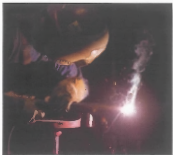
A welder working on environmental upgrades at Jeffrey Energy Center.
