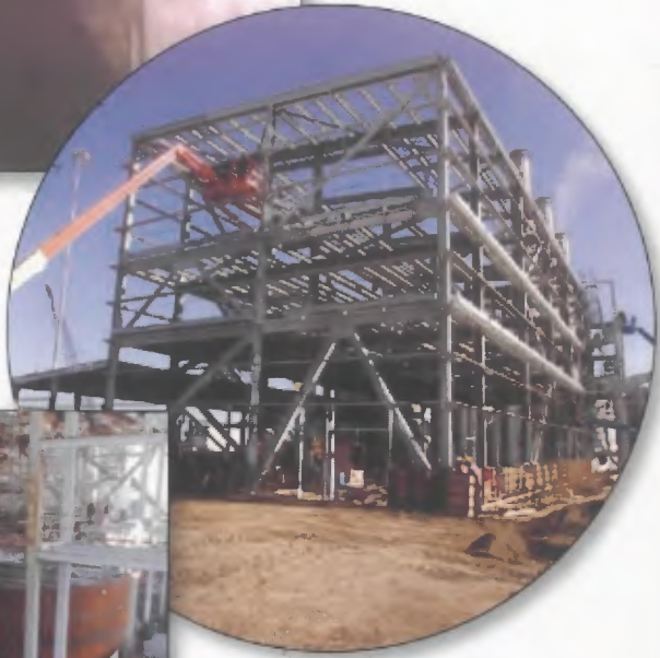
Contractors work on the scrubber dewatering building at Jeffrey Energy Center.
