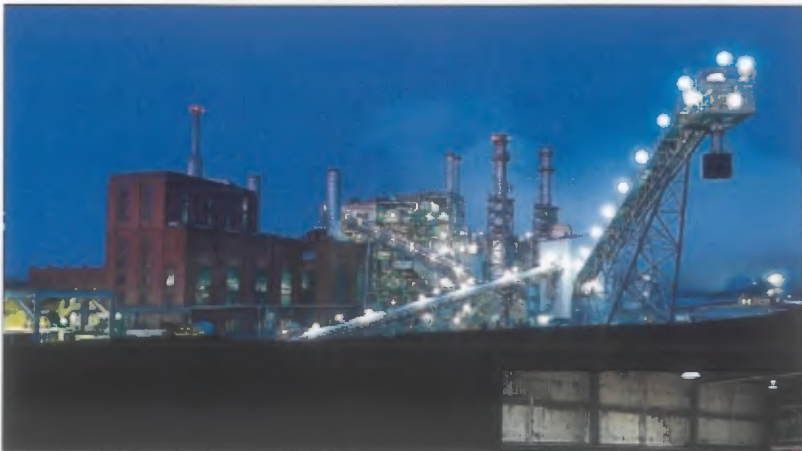
A night view of Tecumseh Energy Center.
