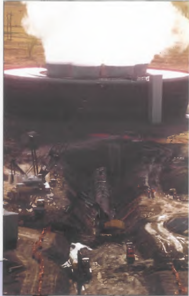
Circulating water line replacement work on unit 3 at Jeffrey Energy Center.
